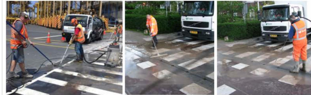
Using a water blaster
