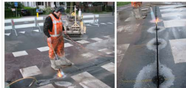
Drying with a torch
